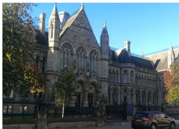
THE ARKWRIGHT BUILDING, NTU.
